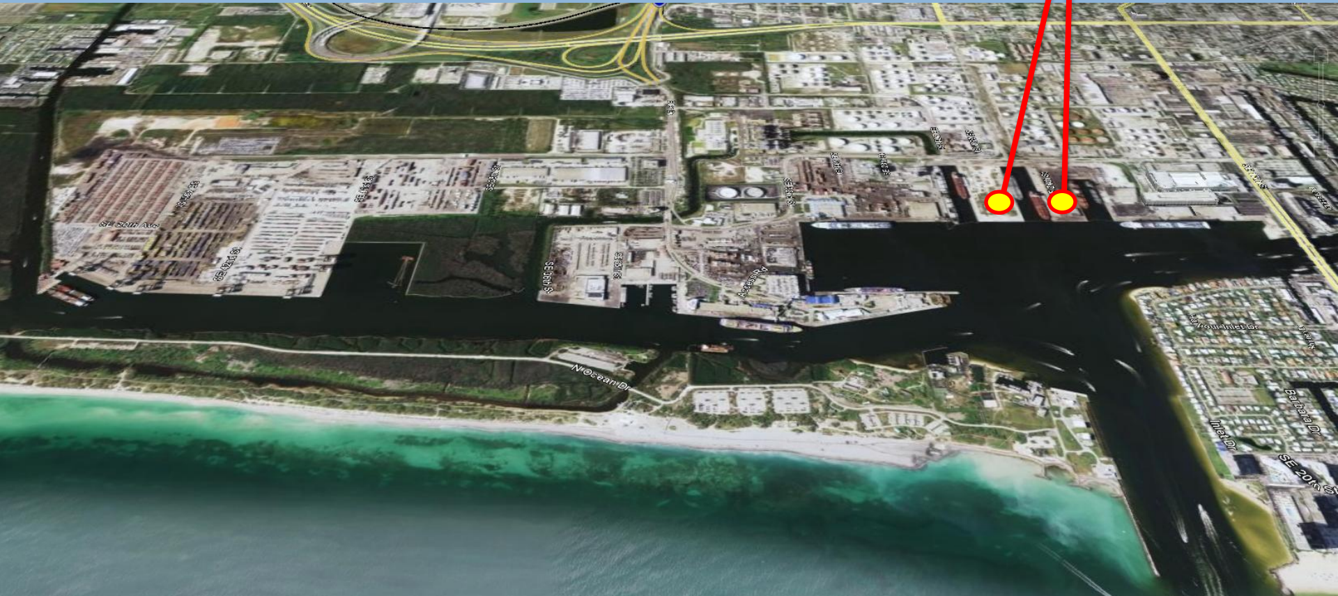
Bulkhead Reconstruction to accommodate larger Vessels
