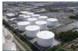
New Vecenergy terminal being built at Port Everglades.
