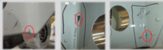
Wing Damage Without Guards
